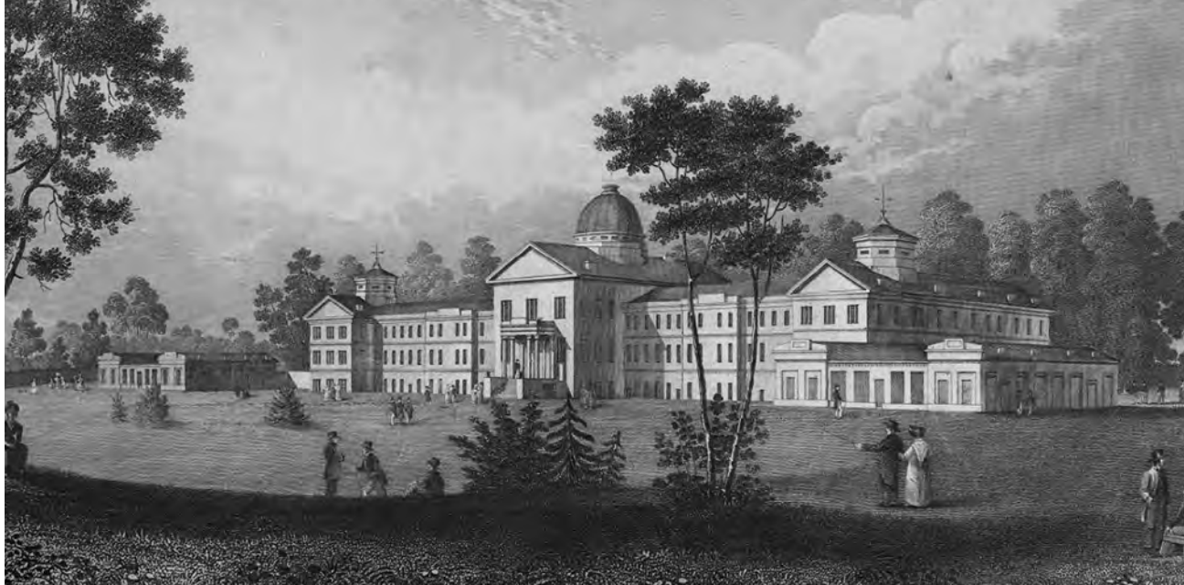
FIGURE 6. Detail of South East View of the Pennsylvania Hospital, Philadelphia , engraving by John G. Exilius, 1814. Library of Congress, Prints and Photographs Division, loc.gov/item/2003666919
