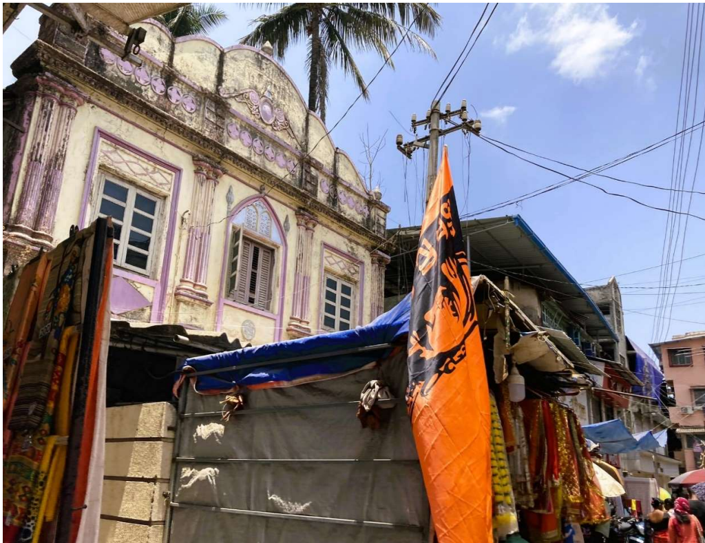
The façade of Beth-Ha-Elohim Synagogue from the Market Street, 2022
