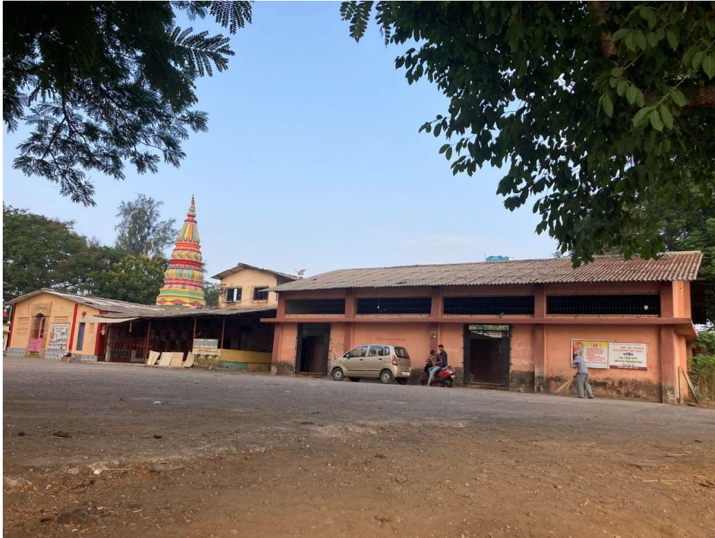
Entrance to the Indoor Unhere Hot Water Springs, Pali, 2022
