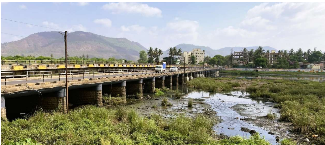
Bridge over Kundalika River Connecting the Villages of Roha and Ashtami, 2022
