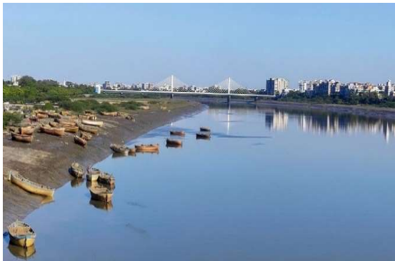
Tapti River- Cable Bridge - Surat
