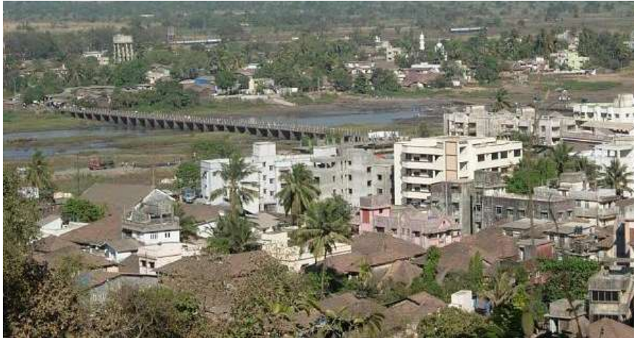
Roha- Bridge Connecting to Ashtami
