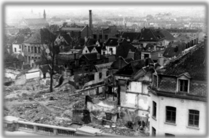
Brussels Palais de Justice, damage from German bombs - 8 November 1944
