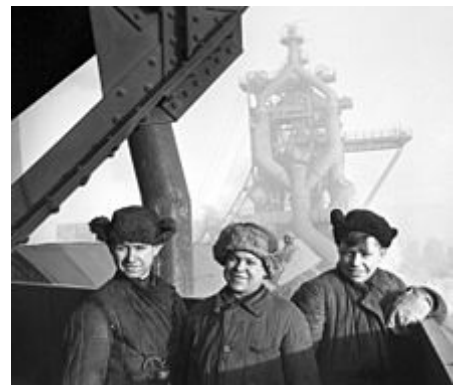
Komsomol members at the construction of blast furnace No. 6 MMK , 1943
