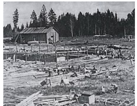
Start of construction of the processing plant Sredneuralsky Copper Smelter (SUMZ) , 1935.
