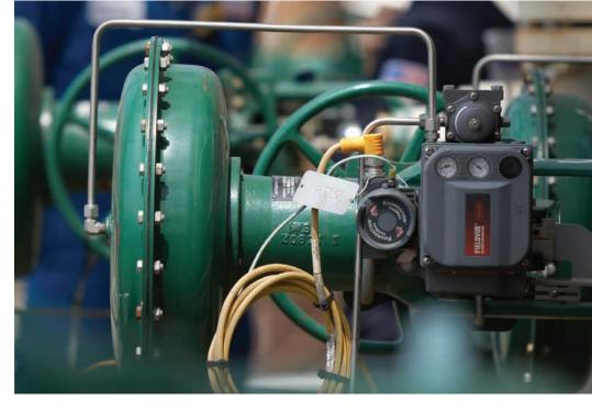
"Valves operating with a digital valve controller and connected to a plant-wide network can generate vast amounts of health and performance data."
